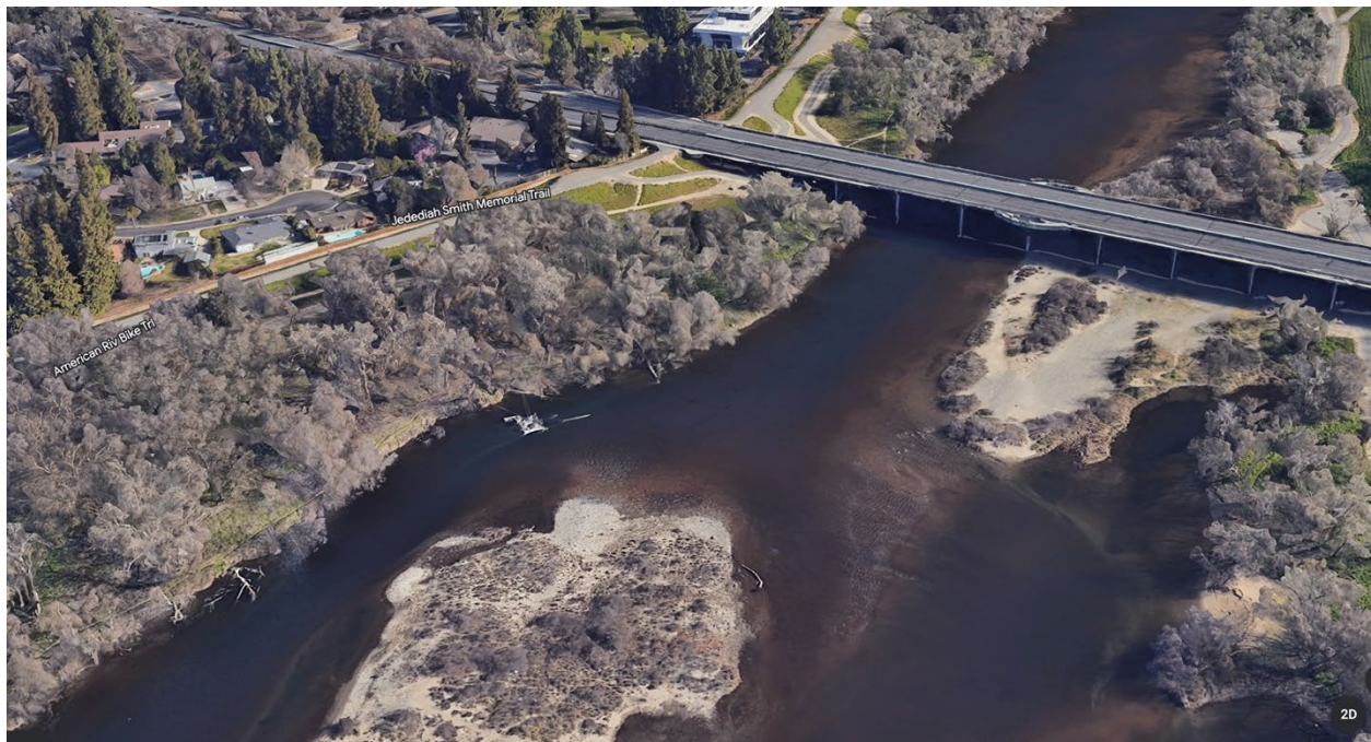
Figure 17: Heavy riparian forest adjacent to Watt Ave Bridge has encampments, is a priority for targeted weed-eating. (Map Imagery ©2023 Google, Landsat/Copernicus)
