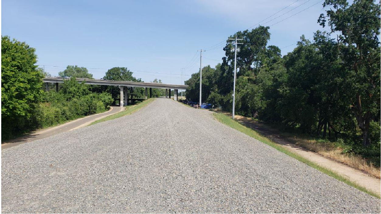
Figure 5: Flood control levees serve as substantial, permanent fuel breaks throughout much of the Parkway. (Image ©2023 Deer Creek Resources)
